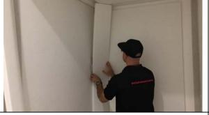
**Step 11:** Place the corner traps on 45° as shown, tuck into the side of the front wall additional 25mm AUTEX panel support
