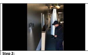
Carry panel with one hand underneathe and one hand on the side
