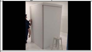
**Step 10:**Some wall adjustment is needed until the ceiling/roof locks in square and tight.
