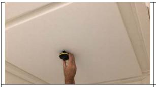
**Step 13:** Place supplied LED light onto ceiling velcro mount
