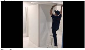
**Step 9:**One person will need to move inside to help place the ceiling/roof into place.
